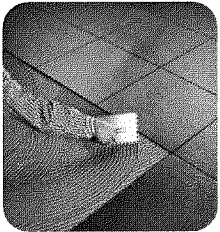
Tile & Stone Installations
